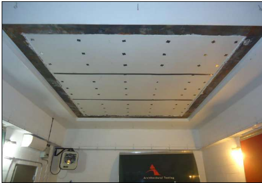
Receive Room View of Test Specimen Installation
